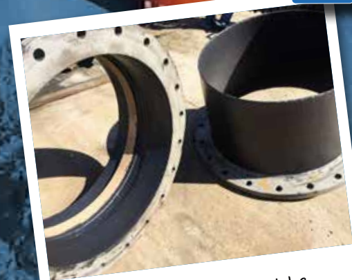
Repair of an expansion tube
